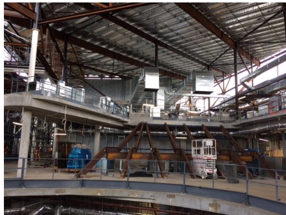
Library amphitheatre steelwork leading from level one up to the mezzanine on level 2.
